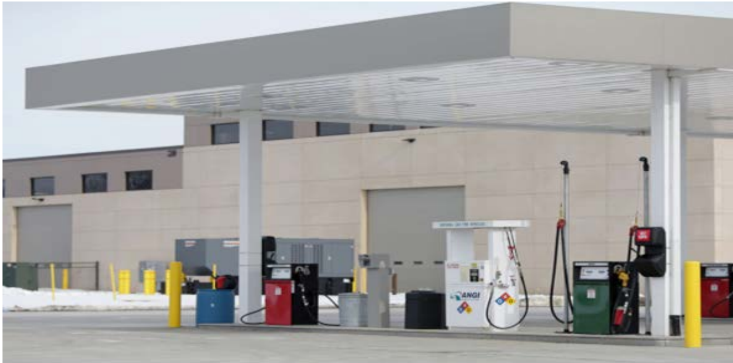
Renewable CNG Filling Station
